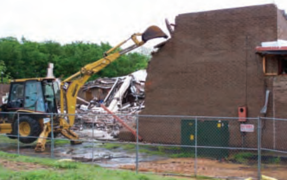
The remaining portion of the academy building being removed.
